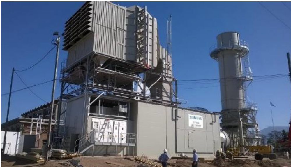
08/31/16 – New Siemens SGT-800 installed on site
